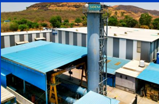
Figure 4. Large water flow calibration facility based on tower volume.
