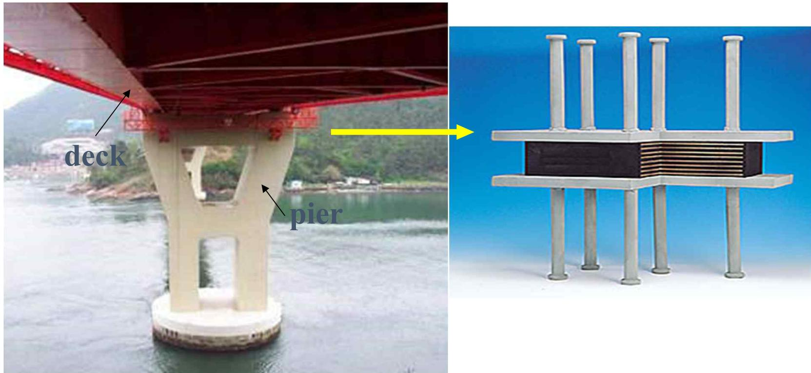
**Elastomeric bearing** used between deck and pier provides a flexibility of bridge against forces caused by earthquake and passage of vehicle on the bridge.
