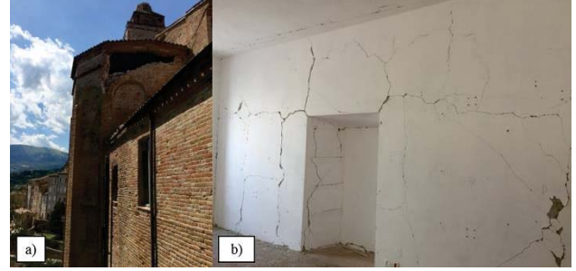
Fig. 3 External cracks on bell-tower and apse a), internal cracks on a wall of the cloister b)
