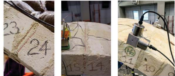
Fig. 4. The three crack hinges.
