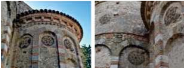
Fig. 4 - Apses details: pilasters and windows
