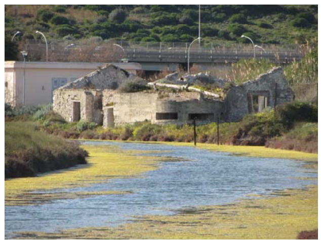
Fig.13. Bunker incorporated in a nineteenth century building to control waterways and road that connected in the 1940s Quartu Sant'Elena to Cagliari - sector 4
