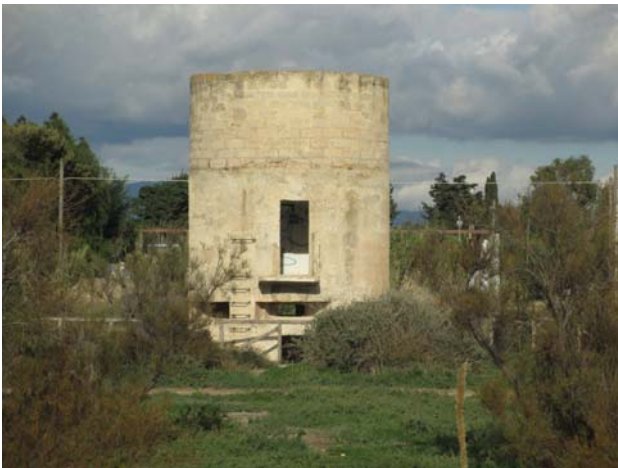
Fig.9. Bunker as a cylindrical water tank - sector 3
