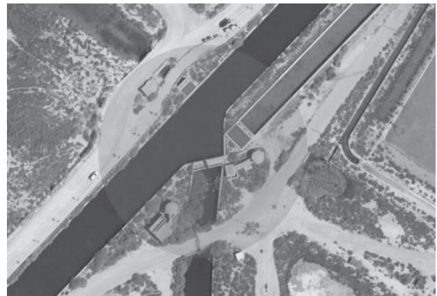
Fig. 15. Bunker located in the sector 2
