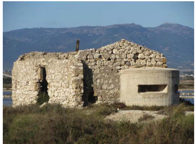
Fig.12. Bunker incorporated in a building - sector 1
