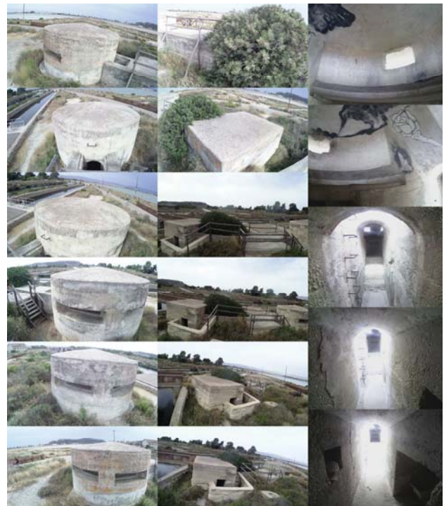
Fig. 16. Photographic survey– sector2
