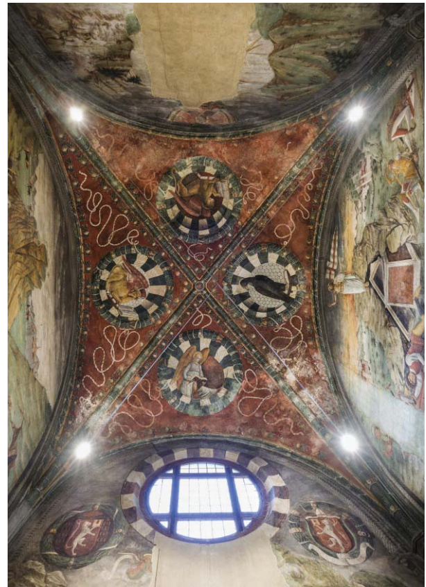
Fig. 1 Intrados of the vault of the Castiglioni Chapel and evident deterioration of the wall frescoes.
