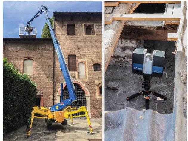
Fig. 5 Spider lift elevator platform used to access the extrados of the chapel vault.
