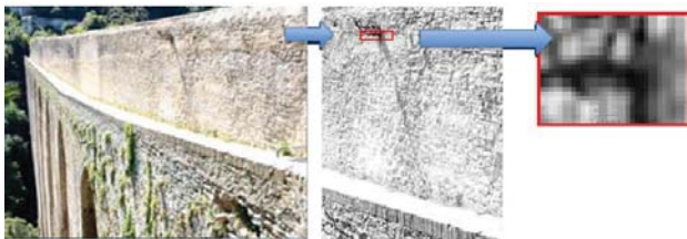
Fig. 7. Camera viewpoint (left) and detail zoom of analyzed Region Of Interest (ROI)(right).
