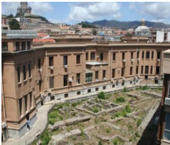
Fig. 6. Courtyard of "Palazzo Zanca", Messina, Italy [22].
