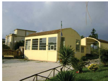
Fig. 4. Vault building n.8
