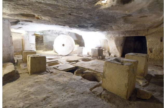
Fig. 3. Hypogeum oil mill of Melpignano: internal view.
