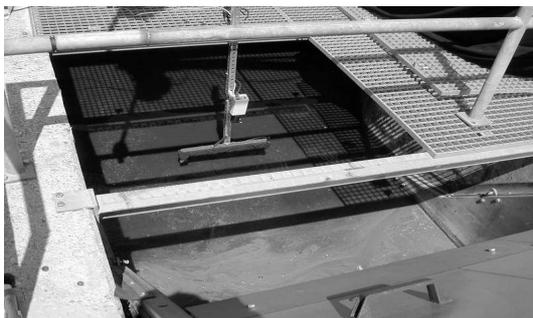
Fig. 10. Measuring system installed above the wastewater flow
